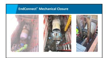
Service Connections – Three Schools of Thought Involves open-cut excavation and installation Excavated of new mechanical connections at each service. Plug and drill method whereby liner adheres to Adhesive host pipe and service corporation Utilizing a robot to mechanically reinstate the Mechanical service corporation.
